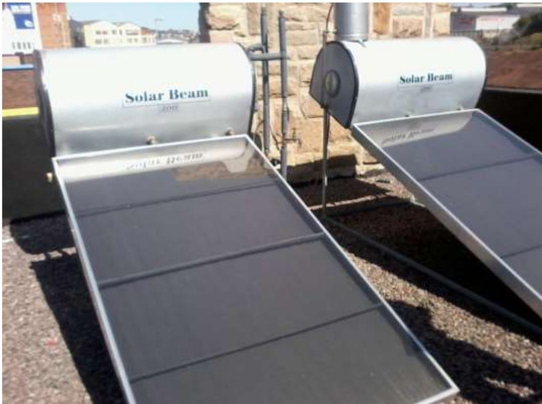
**Figure 6: The new frost resistant flat plate solar water heater designed by Solar Beam (Picture: Margaret McKenzie)**
